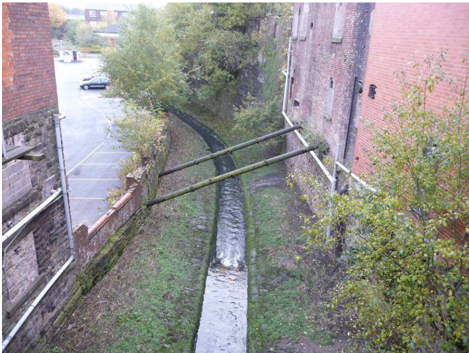
Plate 16 – View downstream from Manor Street bridge
