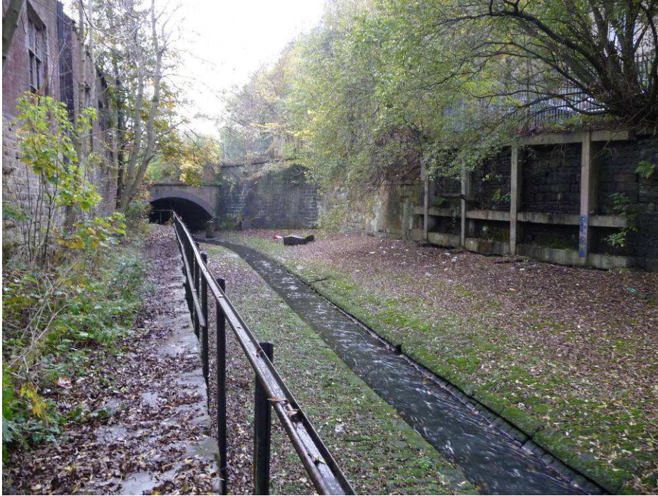
Plate 19 – View downstream adjacent to UU pumping station
