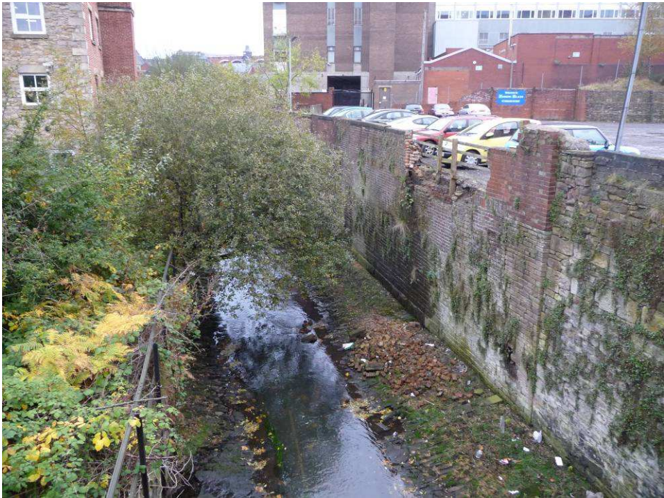
Plate 10 - View downstream from St Edmund Street bridge
