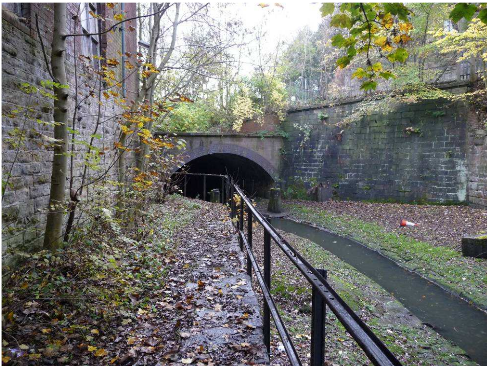
Plate 20 – View downstream to culvert under Church Bank
