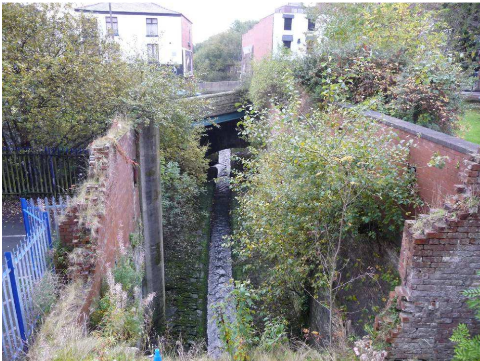
Plate 14 - View downstream from Crown Street bridge
