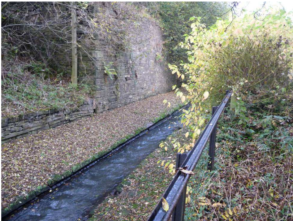
Plate 18 – View upstream adjacent to UU pumping station
