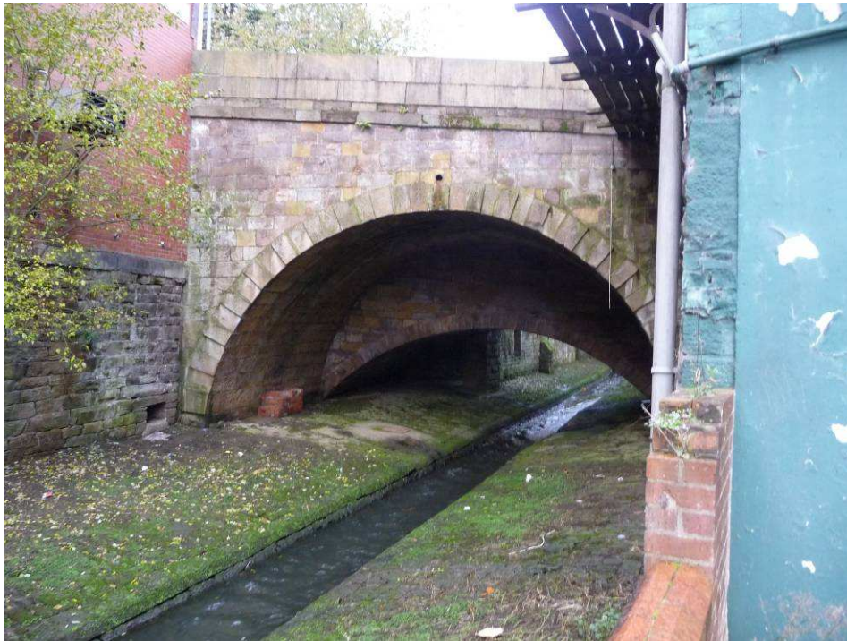
Plate 17 – View upstream of Manor Street bridge
