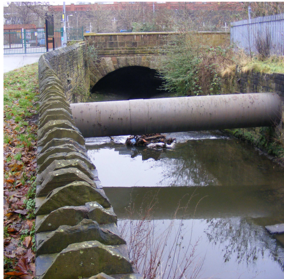
Plate 6-1: Trunk Sewer upstream of Chorley Street Bridge
