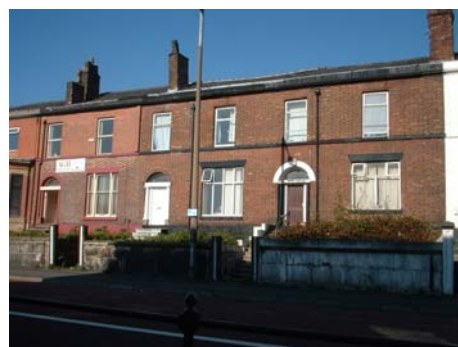
Figure 17 Terraced properties western end of St George's Rd
