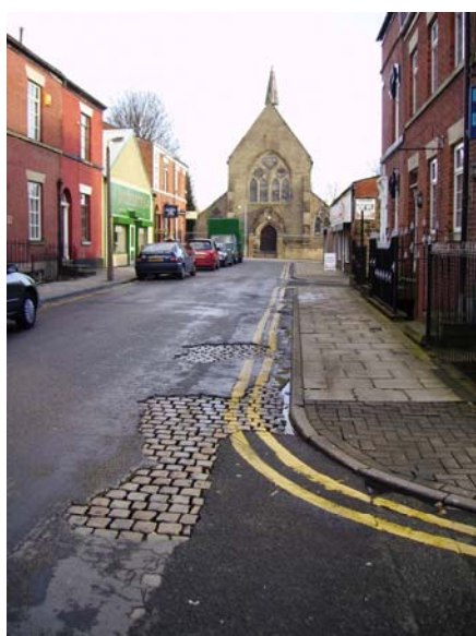
Figure 16 Setts visible under tarmacadam in Bark St East
