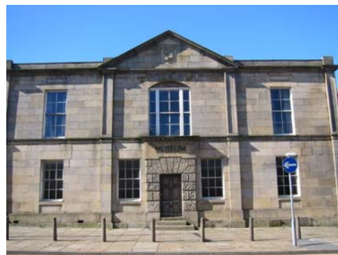
Figure 3 Little Bolton Old Town Hall
