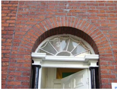
Figure 12 Fanlight on Bark Street East
