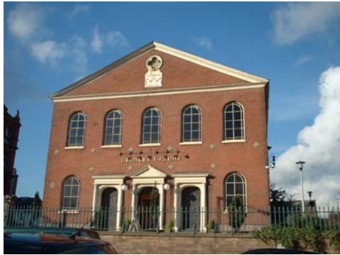
Figure 8 Former Wesleyan Chapel (now Stanley Casino)
