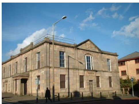
Figure 10 Little Bolton Old Town Hall
