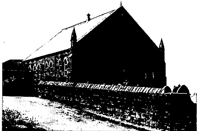
Figure 4. Tootington Road Methodist Church
