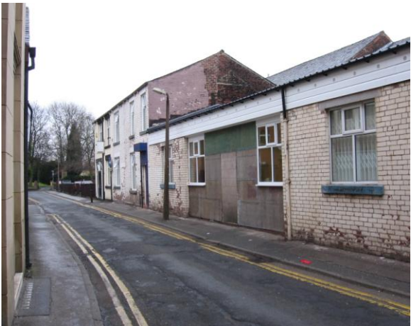
Fig.19: The south side of Princess Street, from the west
