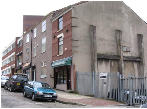
Fig.18: The north side of Church Bank
