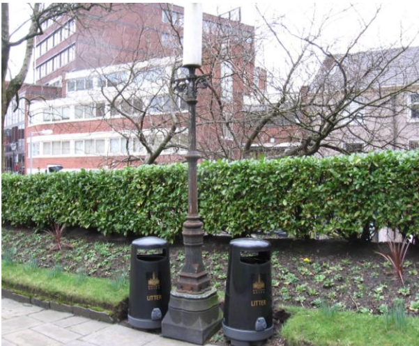
Fig.14: Victorian cast-iron lighting column in the Church yard, with incompatible post-war lamp, and plastic bins.
