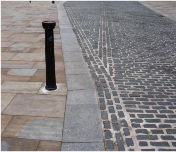
Fig.13: High quality natural paving and setts, with a traditional-style bollard on Churchgate
