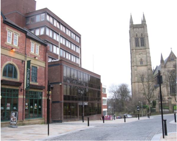
Fig.6: Travel House, an office building constructed in 1974, with the late 1990s Varsity pub to the left, and the church beyond.
