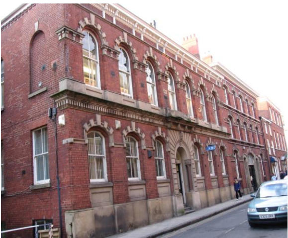
Fig.4: No.28 Mawdsley Street, former Poor Law office building, built in 1865
