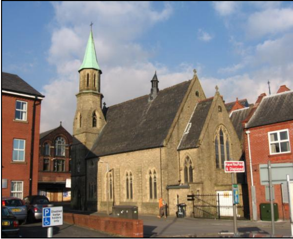
Fig.24: St Patrick's Church, Great Moor Street, seen from the south-west
