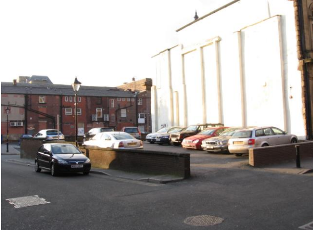
Fig.23: the corner gap site south of the former County Court, on Cheapside Square
