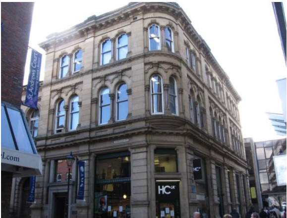
Fig.7: the Bridgeman Buildings on Exchange Street, refurbished in 1990 for retail use.
