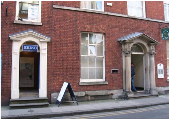
Fig.1: Former town houses on Mawdsley Street retain original doors with pediments
