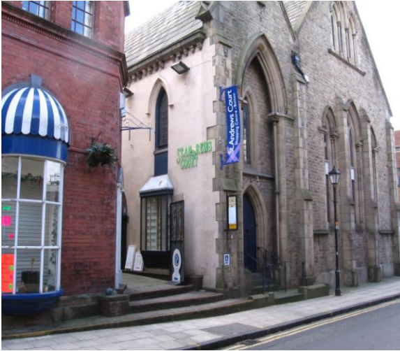
Fig.5: Former St Andrew's Church built in 1846 as a Presbyterian chapel and converted to retail use in the 1980s.
