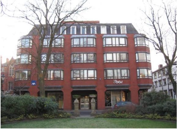
Fig.6: Provincial House, built in 1974 on the site of the former infirmary
