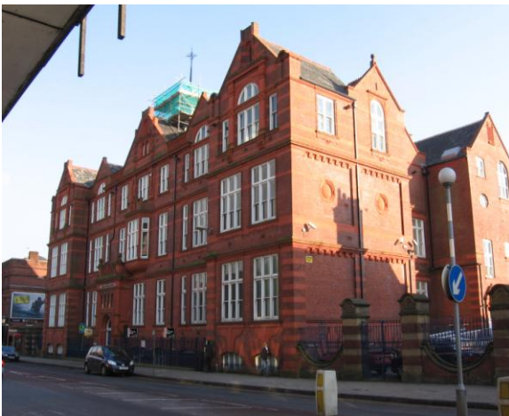
Fig.26: Former school on Great Moor Street
