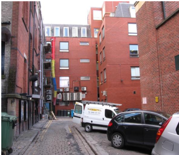
Fig.22: Looking north on Chancery Lane, the rear of Provincial House was built across the line of the street in the 1970s,.
