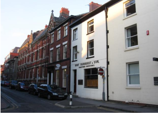
Fig.18: A mixture of brick and render on the south east side of Mawdsley Street
