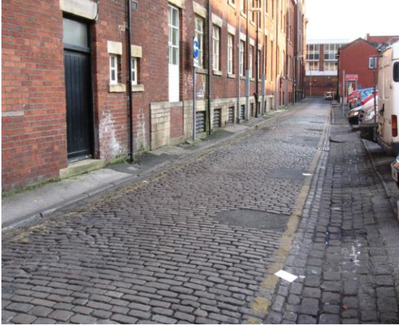
Fig.19: traditional stone setts, granite kerbs and gully treatment on Back Mawdsley Street
