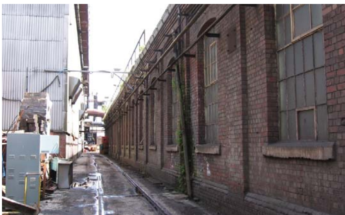
Figs 30 and 31: enlarged opening in a gable-end of the erecting shop, and view with rail tracks along the narrow access between the mechanised foundry and the small workshops.
