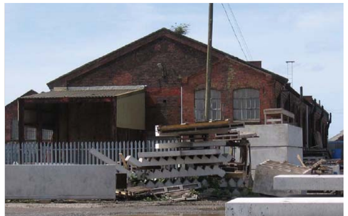
Figs 17 and 18: North elevation of paint shop and south gable of spring smithy
