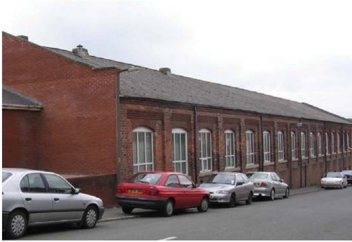
Figs 13 and 14: The tube shop from the south and the dining room on Gooch Street
