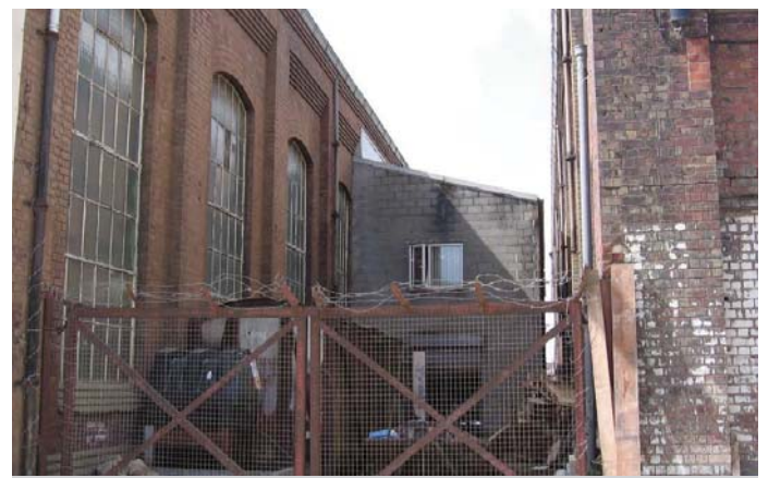
Figs 26 and 27: Lean-to addition to west side of erecting shop, and infill adjacent to heavy machine shop
