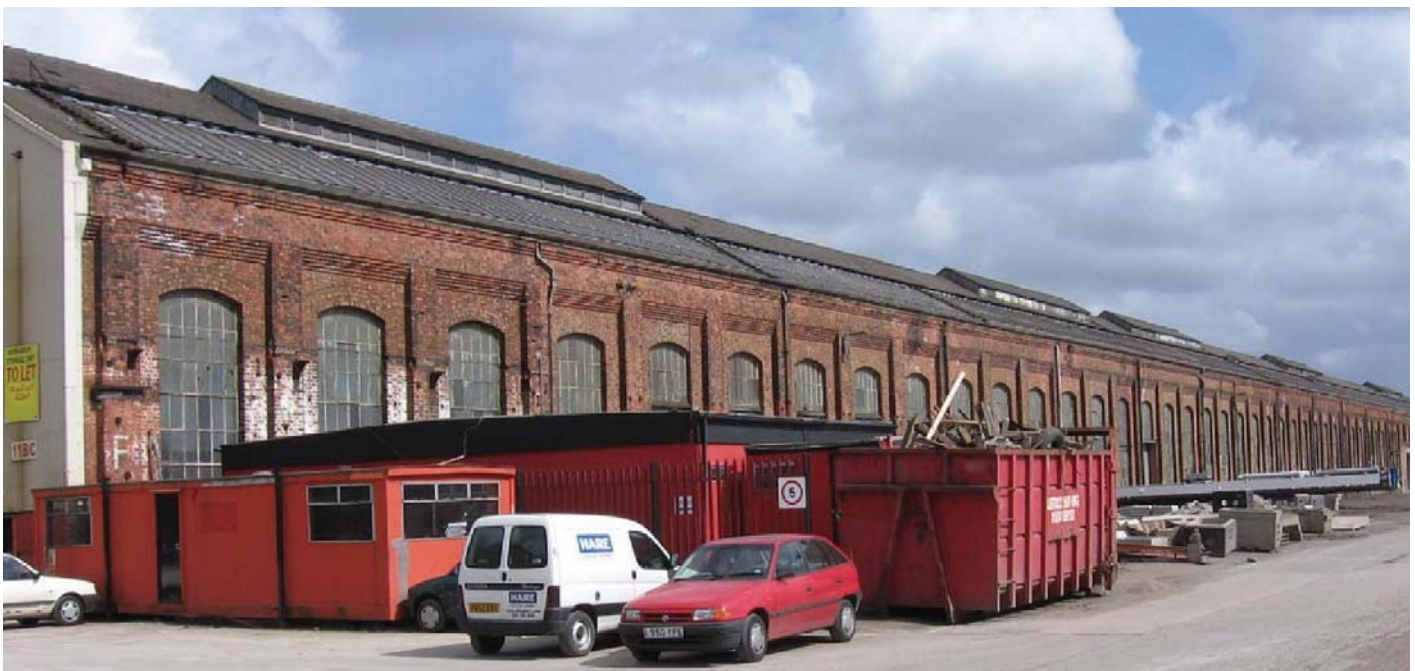
Fig 1: View of the southern section of the former erecting shop from the north-west; the pale cladding to the left gable marks the demolition of a central section
