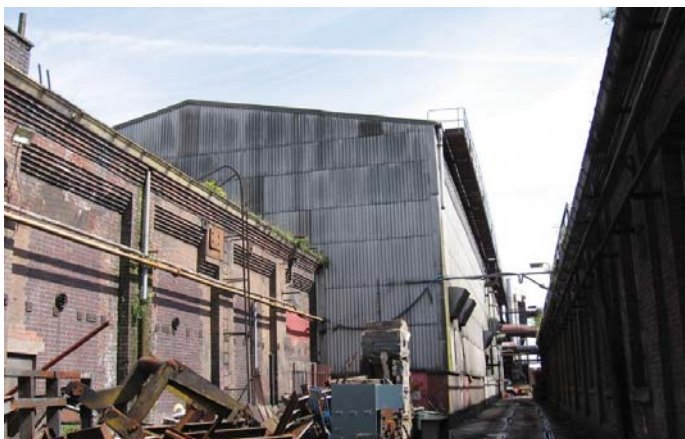
Figs 24 and 25: Mechanised foundry cupola on above, portal frame shed below
