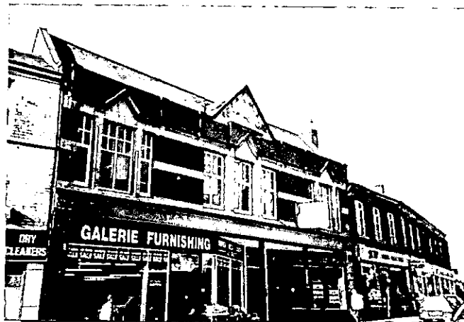
Figure 14. Co-op New Central Store
