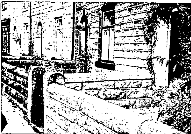
Figure 7. Dressed stone walls Lee Lane
