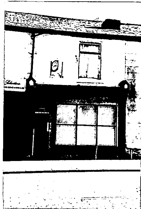
Figure 24 Shop front in need of repair
