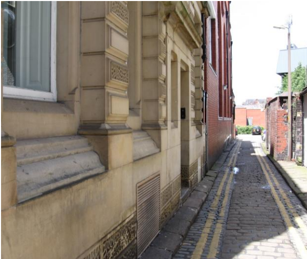
Fig.19: historic stone setts and kerbs on Woods Court, an alley north of Deansgate
