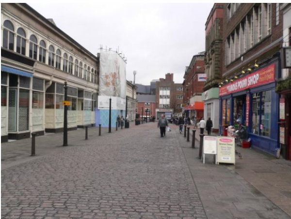
Fig.20: re-laid setts and natural stone paving on Corporation Street, with cast-iron bollards
