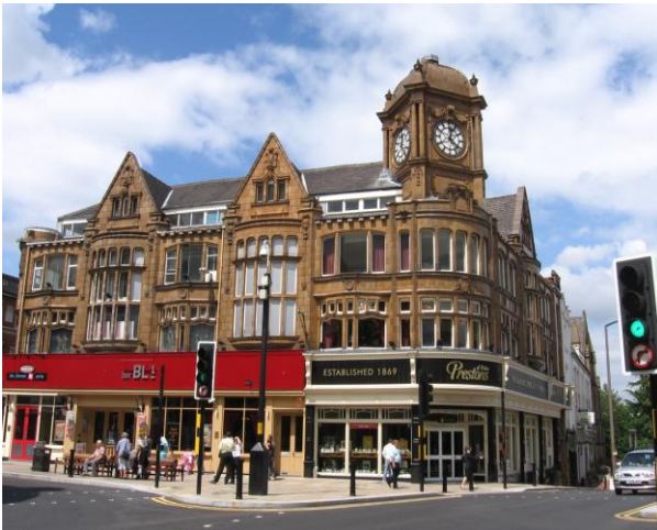
Fig.4: Prestons' jewellery store opened in 1904, with a colourful terracotta and faience frontage (compare with Fig.2)
