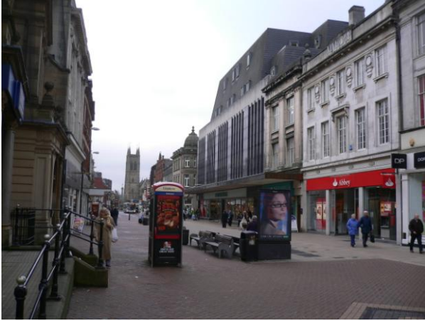
Fig.25: A view eastwards along Deansgate, showing the dominant scale of the mansard roof on the Marks & Spencer building.
