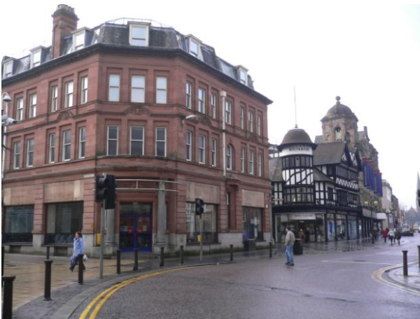
Fig.18: Contrasting materials: red sandstone and black and white half-timbering on adjacent buildings on the south side of Deansgate.
