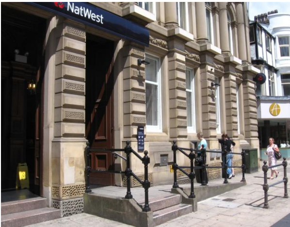
Fig.24: access ramp to a bank on Deansgate
