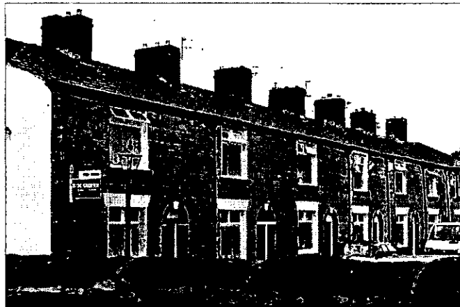
Figure 2. Green Street South Side
