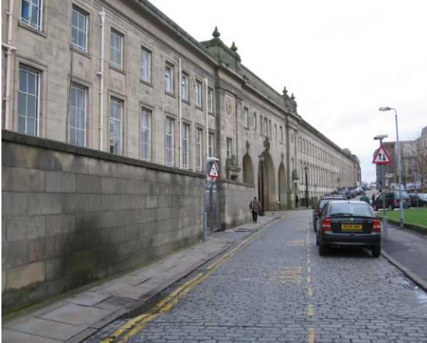
Fig.13: Queen Street and the west front of Le Mans Crescent
