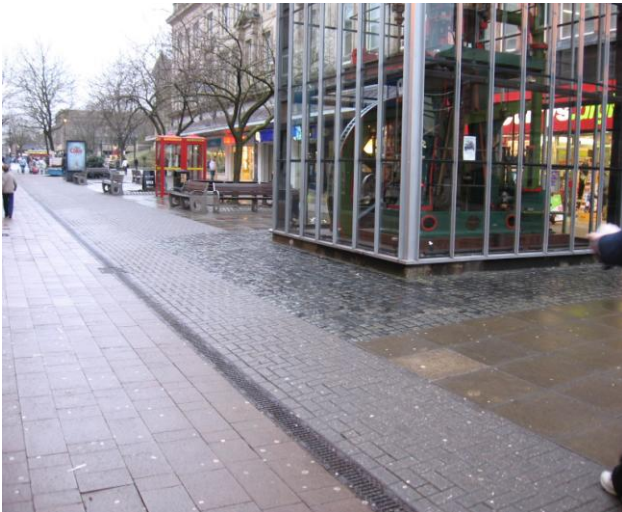
Fig.19: concrete paving surfaces on Oxford Street, now in need of enhancement
