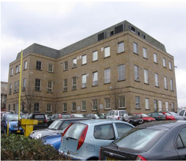
Fig.22: Post-war offices on the east side of Black Horse Street, with large area surface car park.
