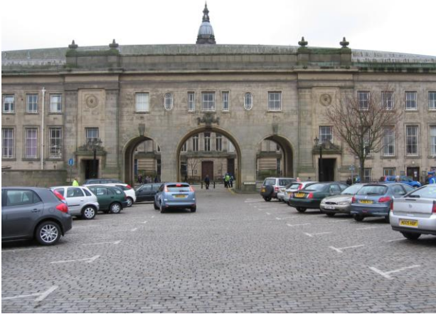
Fig.8: View east along Cheadle Square towards Le Mans Crescent
