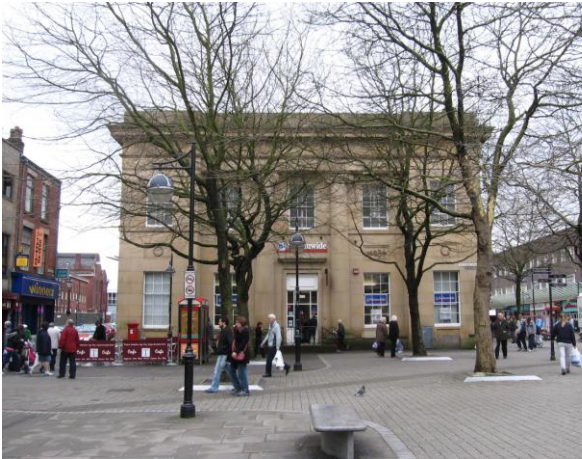
Fig.1: Exchange Buildings, built in 1825
