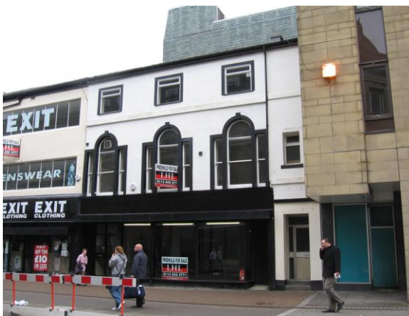
Fig.15: No. 6 Oxford Street retains early 19 th century windows to first floor, although the ground floor shop front is intrusive.
