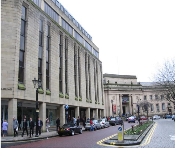
Fig.16: The 1970s Wellsprings Building is faced in sandstone ashlar, to complement The Town Hall.
