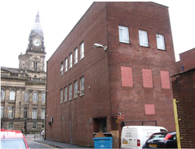
Fig.21: The ugly side elevation of a retail property on Coronation Street, off the south side of Victoria Square, wheeled bins are also intrusive here.
