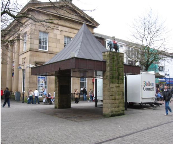
Fig.24: The charity shelter at the north end of Newport Street blocks views down the street and has an unclear function
