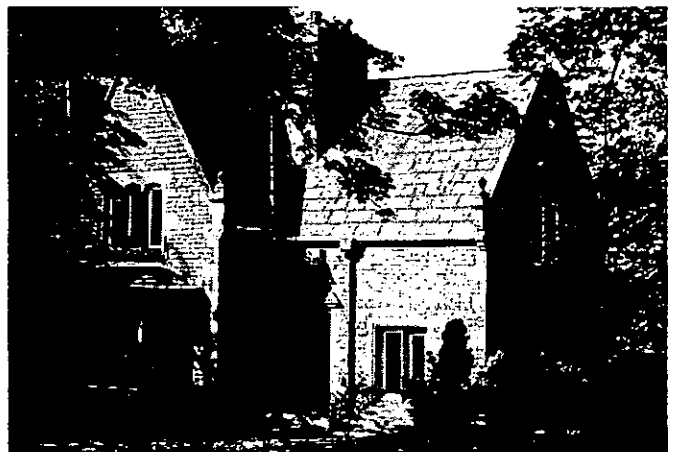
Figure 2. Heaton Grange Gate House, Chorley New Road
