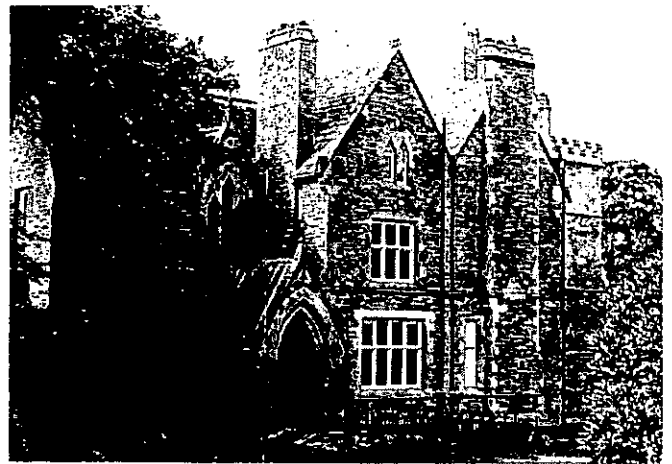
Figure 4. Ladybridge Conference Centre, Chorley New Road
