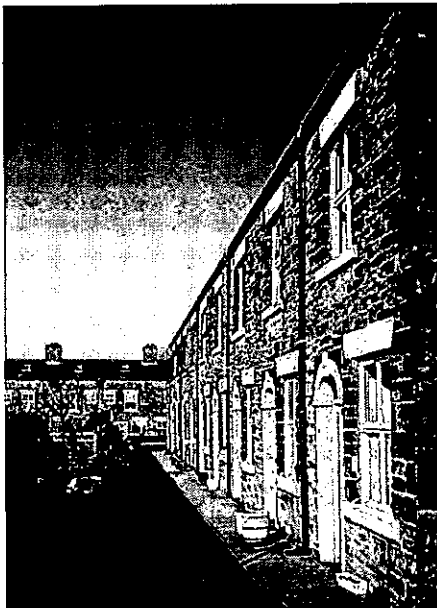
Figure 6. Cottages, Church Street
