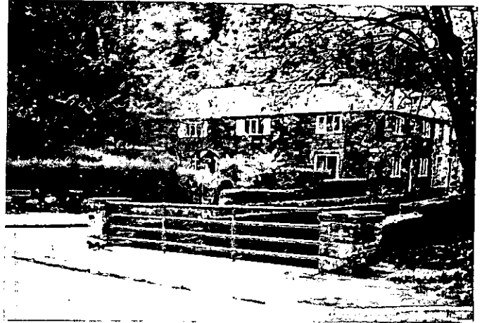
Inappropriate steel bridge at entrance to village
