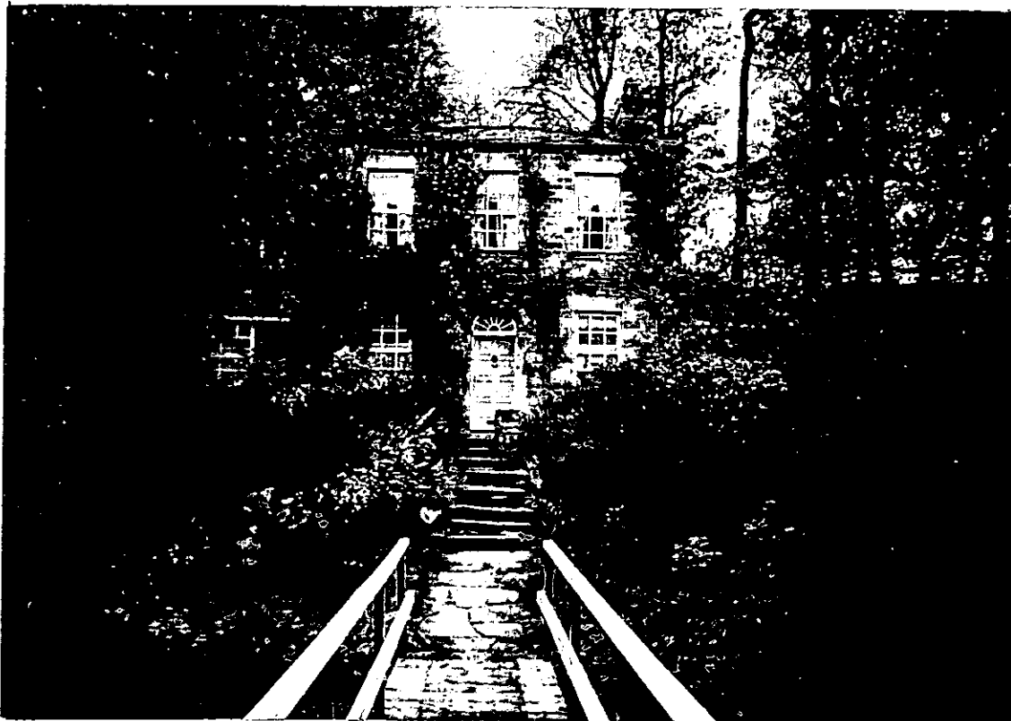
No 75 Barrow Bridge Road
