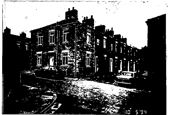
Figure 8. Overseers houses facing Bazley Street
