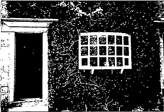
Character is lost where bow windows have been inserted which interrupt the flat facade
