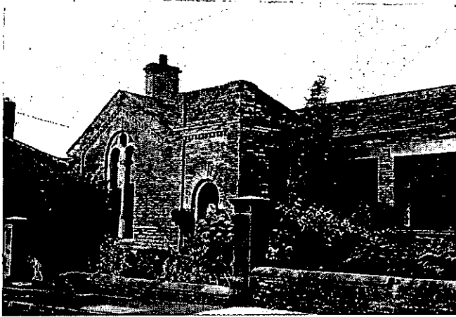
Figure 5. Former school , Ashworth Lane
