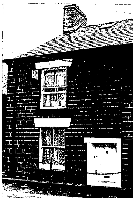
Figure 10 234 Ashworth Lane, Bank Top Traditional door & windows
