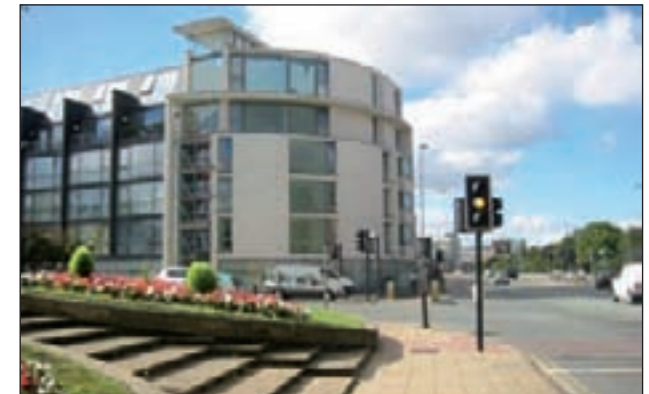
New landmark buildings at junctions.
