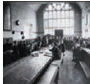
Bolton Grammar School, Undated. The original school building near St Peters Church, shown here, dated from the mid 16 th century and was demolished in the 1880s. The site is now occupied by the Parish Hall, completed 1883
