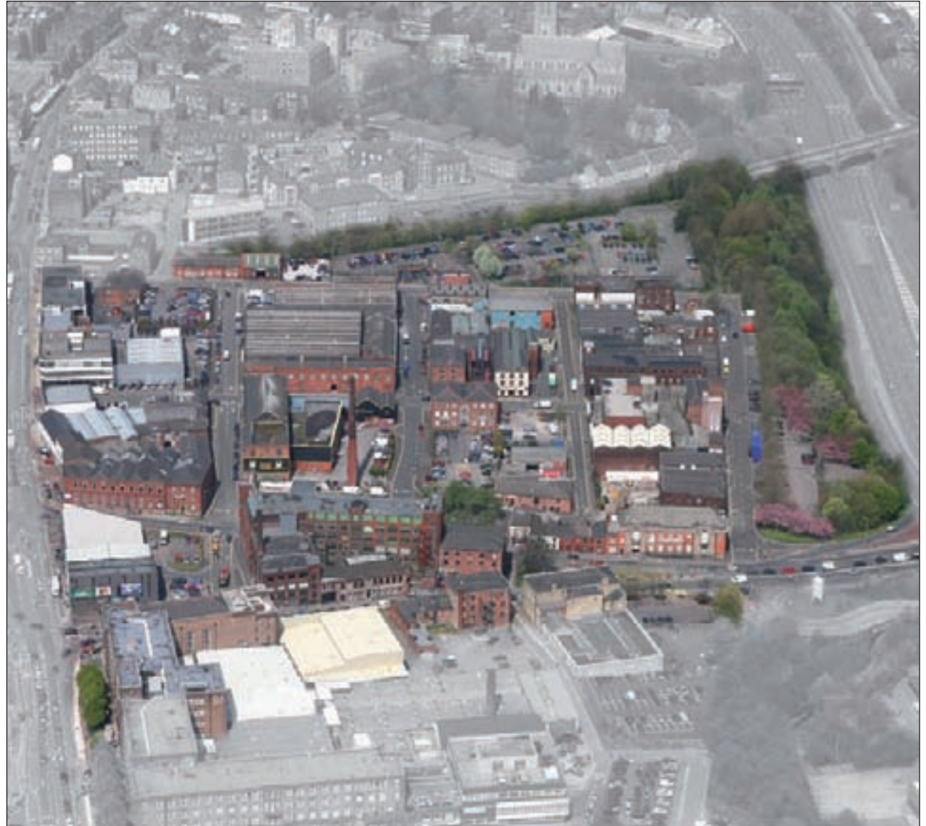
Shiffnall Street / Bridgeman Place from the south.
