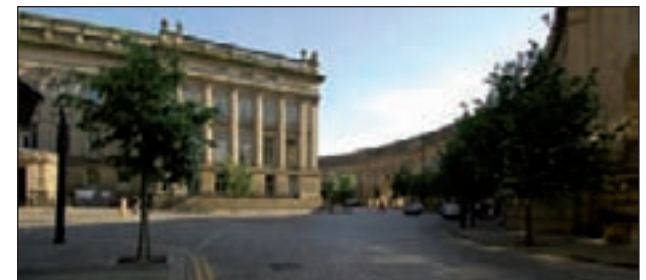
Town Hall and Le Mans Crescent.
