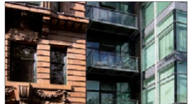
Contrast using materials and facade depth.
