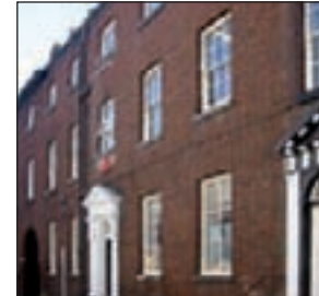
Wood St. The middle class domestic terrace established itself from the late 18th century as the characteristic urban type in St Peters away from the main commercial streets. The reuse of these buildings as offices has helped preserve some of their original character. Note the fine detailing round the doorways.
