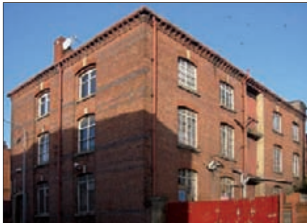
19th century warehouse, Salop Street.
