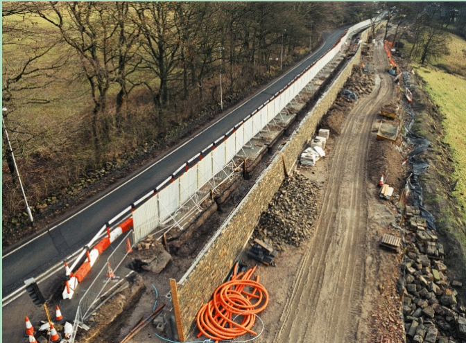
Picture 5.17 Linfitts wall, Delph
