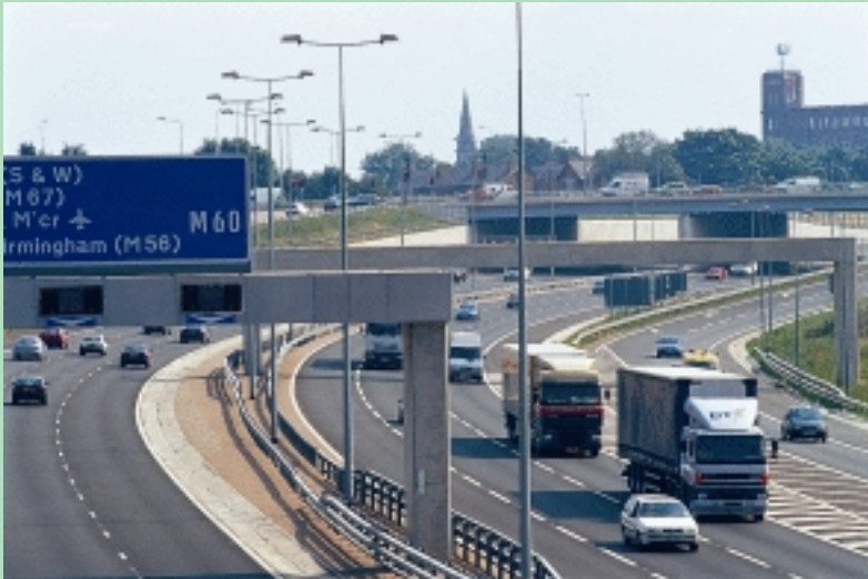
Picture 5.4 M60 motorway
