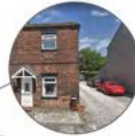
Off street parking provided communally to end of terrace via lane
