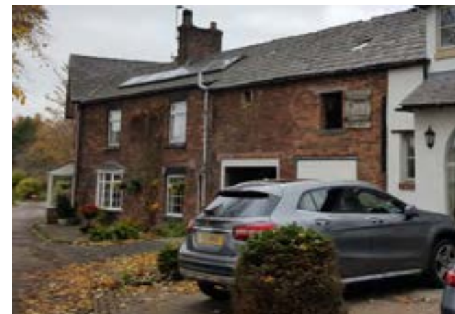
Traditional stonework to corner property.
