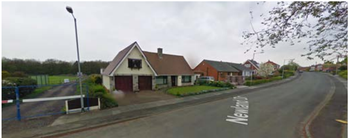
South West corner showing increase in storey height from one to two story moving up the hill towards Manchester Road
