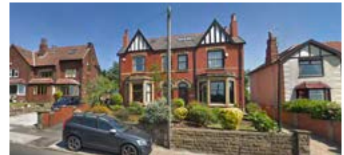
Variety of massing and architectural detailing along Newbrook Road
