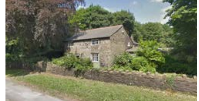
791 and 793 Manchester Rd (grade II listed)
