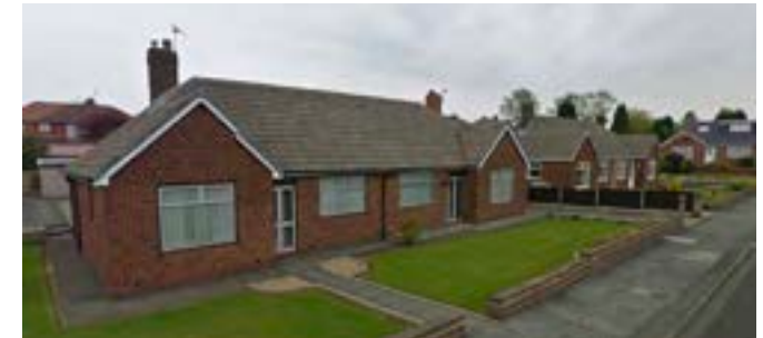
Symmetrical facade with defensible space, defined outlines and prominent chimneys
