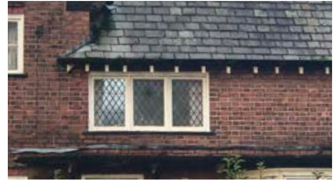
Flemish bond brickwork with burnt headers
