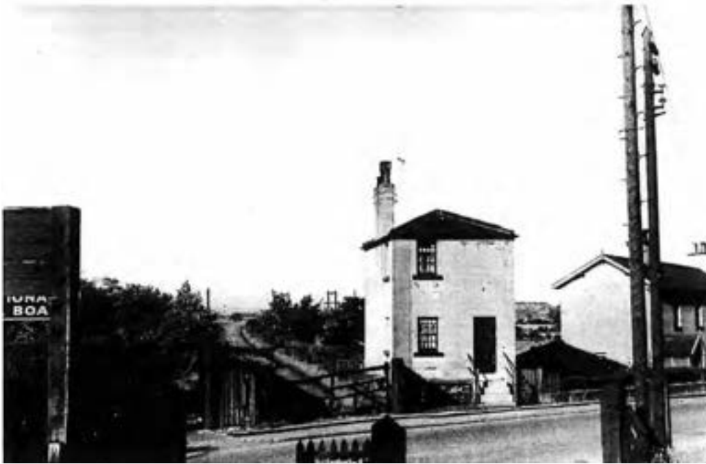
Crossing Keeper's House (photo: Harry Townley)
