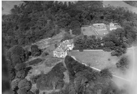
Aerial photo of Hulton Hall
