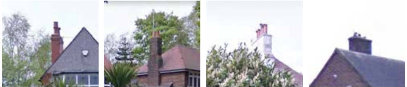
Prominent chimneys throughout this character area
