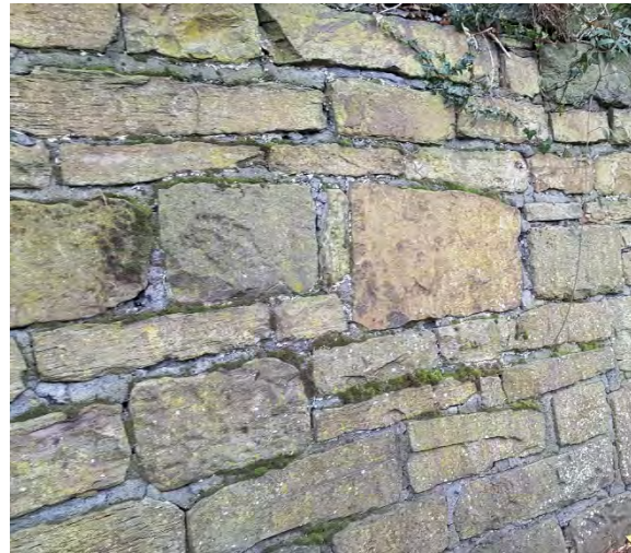
Hulton Park Ha-ha (Slate walling)
