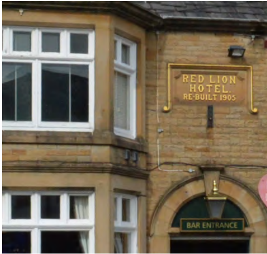
Red Lion Hotel (Limestone and sandstone walls, and slate roofing)
