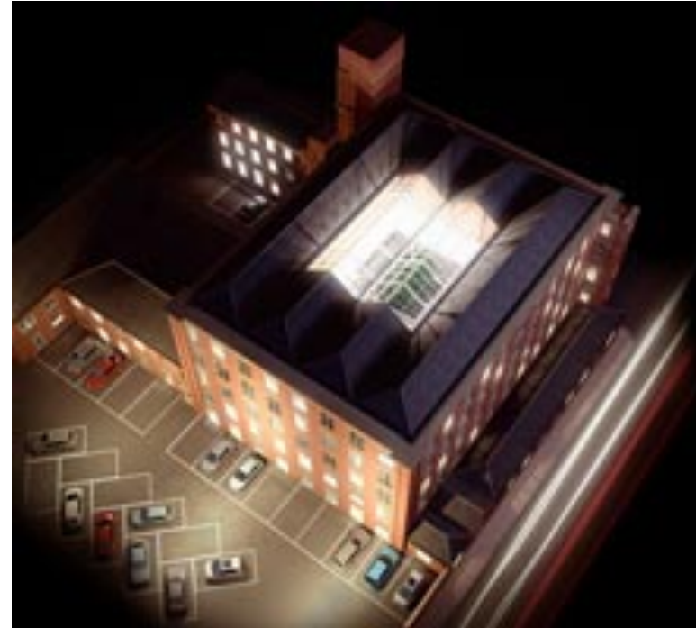
Atlas Mill: 69 apartment residential conversion completed, high quality, energy efficient and affordable prices
