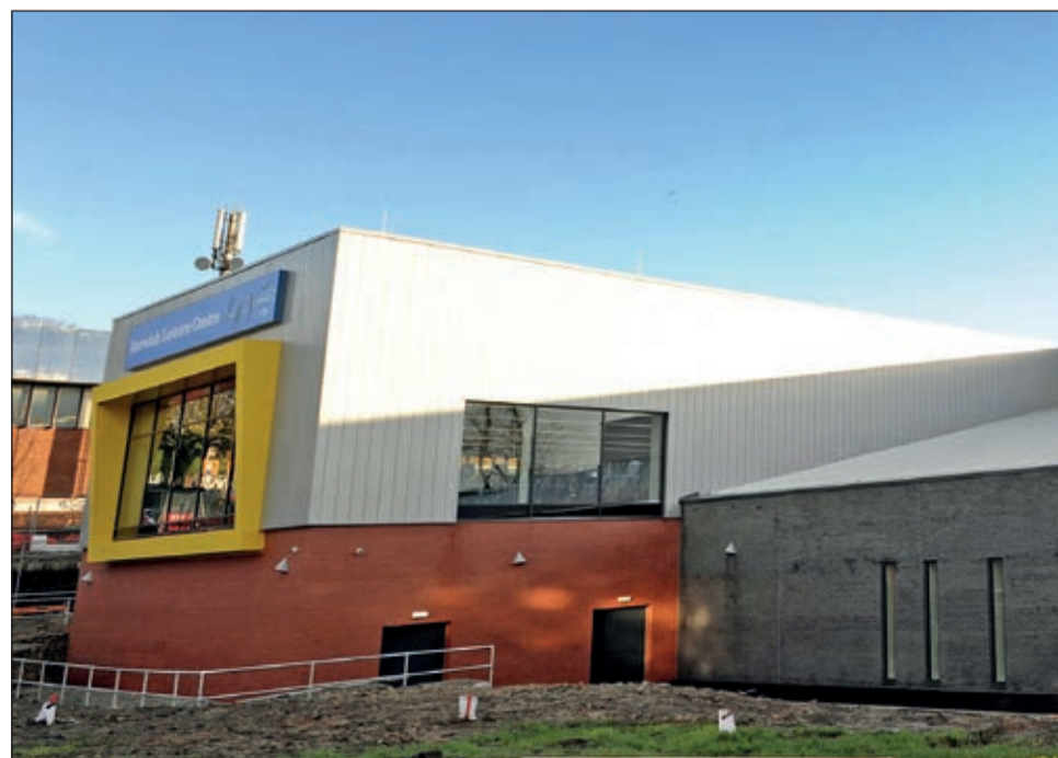
NEW CENTRE: The new facilities at Horwich have now opened
