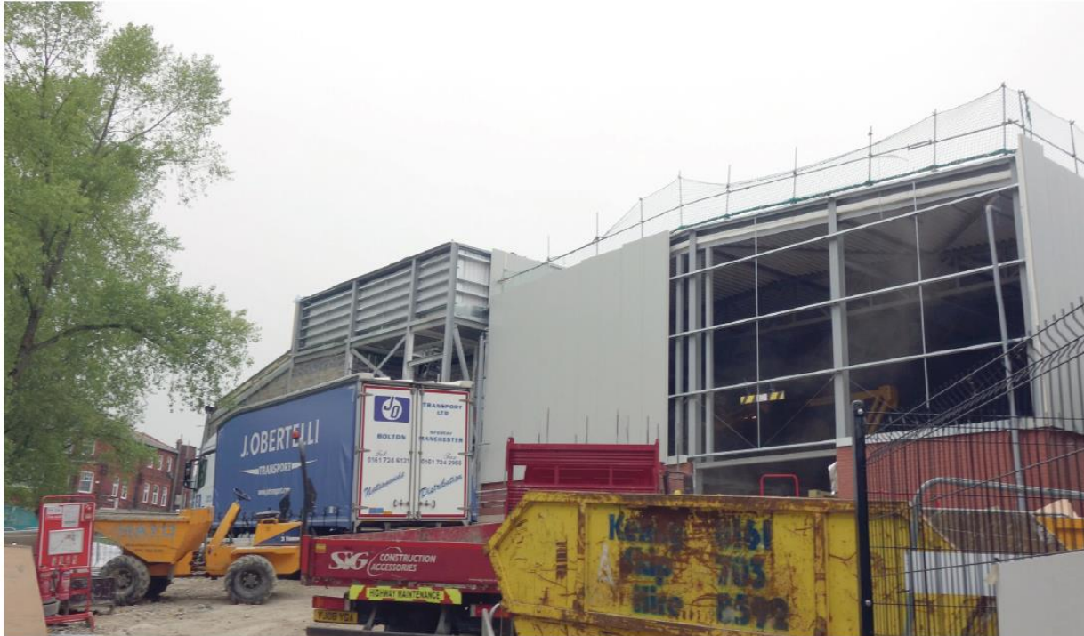
Building works progress at the new leisure centre
