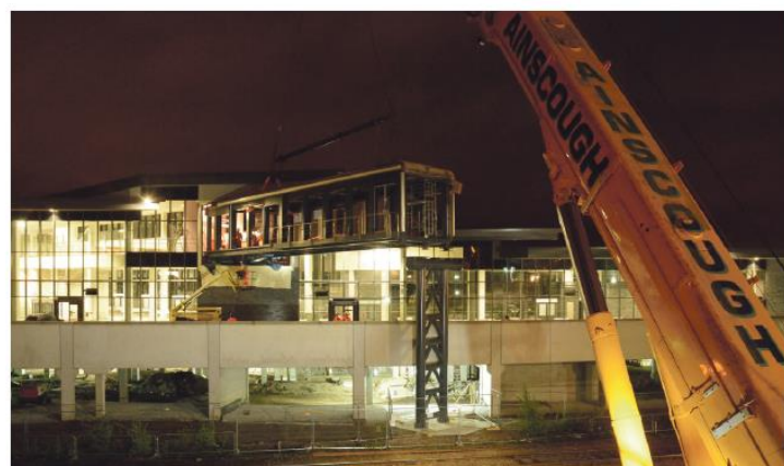
Finishing touches to interchange
