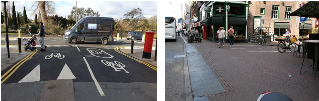
Figure 5: Comparison of the raised table design (left) with a continuous footway (right)
