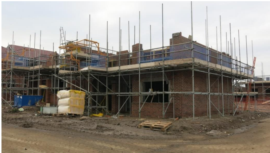
House building on Hill Lane
