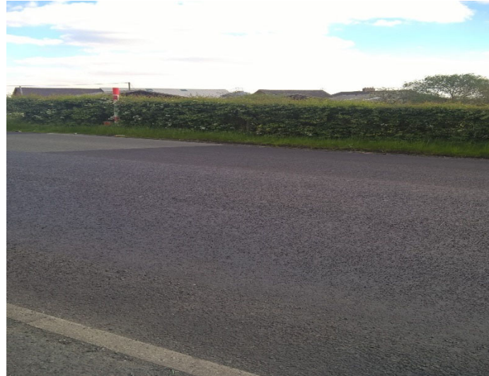
Carriageway patching in preparation for surface treatment
